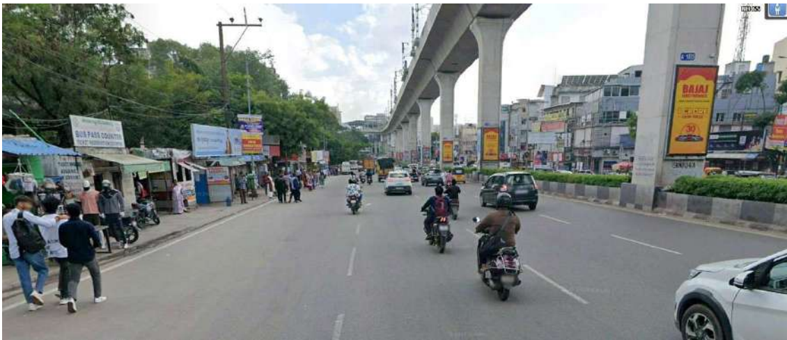
Figure 4-7 NH 65 Site picture
