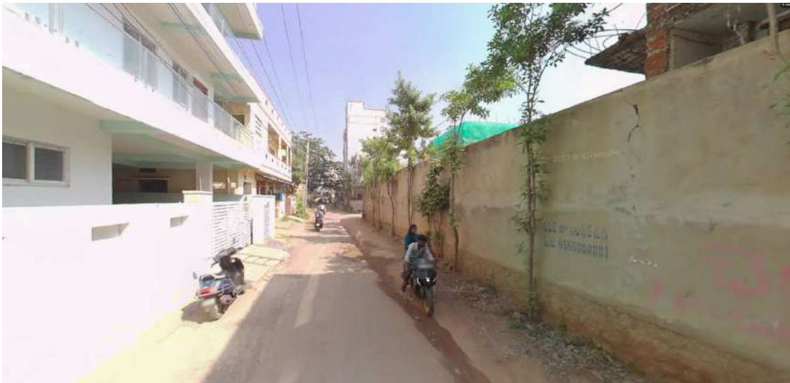
Figure 4-79 Site Photograph of Vijayapuri Colony Road
