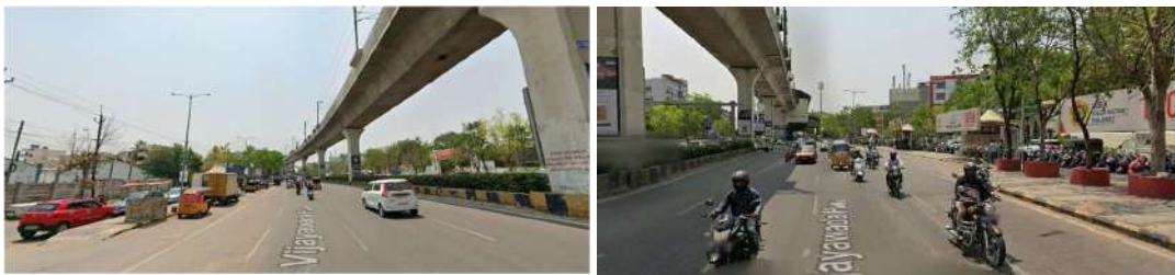
Figure 4-67 Site Photographs of Metro Corridor
