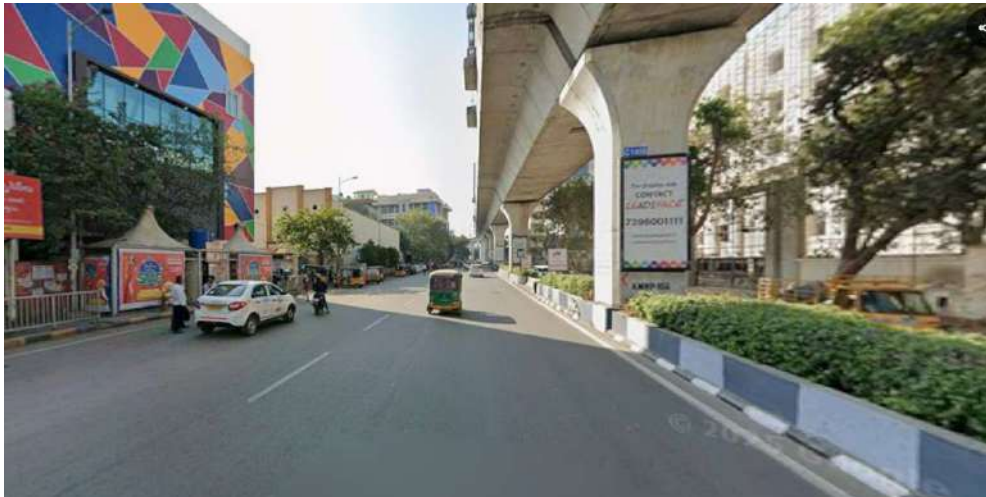
Figure 4-9 Yousufguda road site picture
